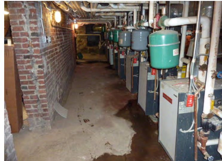
Array of gas-fired hot water boilers is scheduled to be replaced this year with new boilers.
