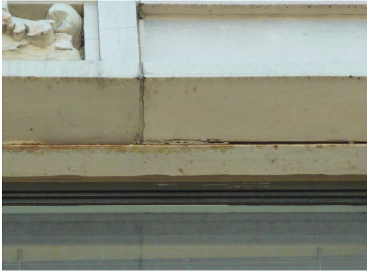
Repair and re-caulking of the limestone ornament on the building facades is shown for Year 1.
