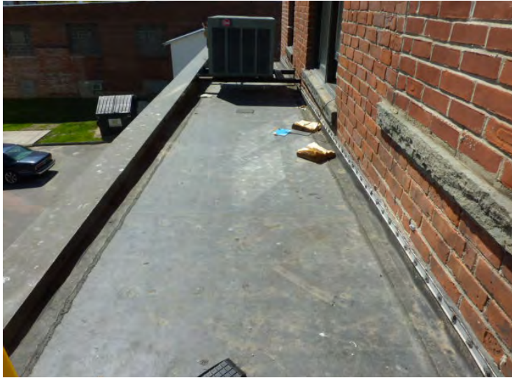
Single ply membrane accessible at the time of our visit appears to be in good condition and is shown in the plan to be replaced in Year 8.
