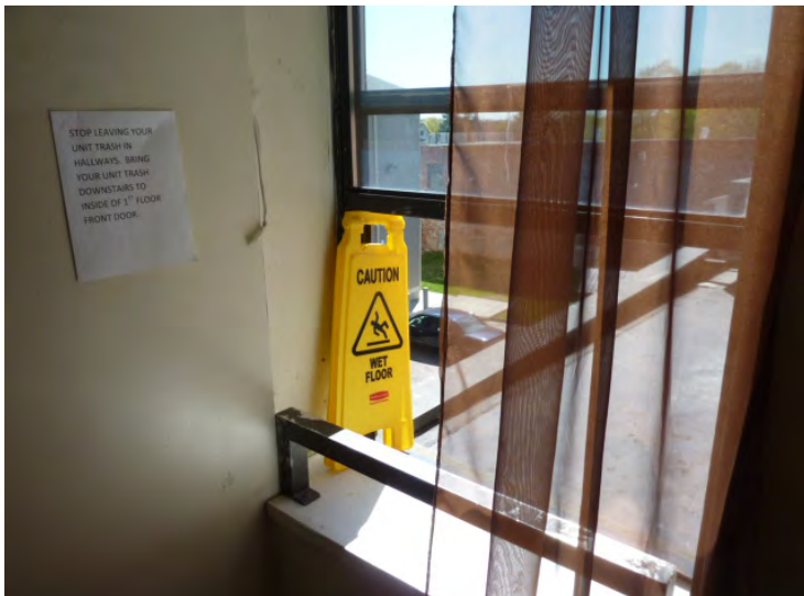
Lower window sash must be propped open or it free falls closed. Window replacement is shown in Year 3 of the plan.
