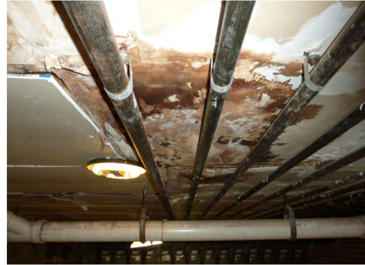
Typical water damage at fire-rated basement ceiling. Rated basement ceiling, walls and doors must be repaired in Year 1.
