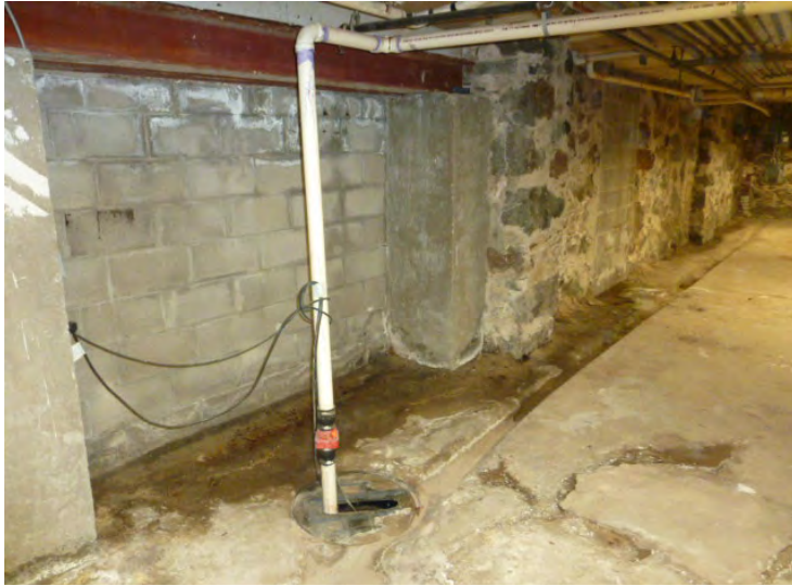
Signs of historic water damage at the building foundations and one of the several active sump pumps in the basement.
