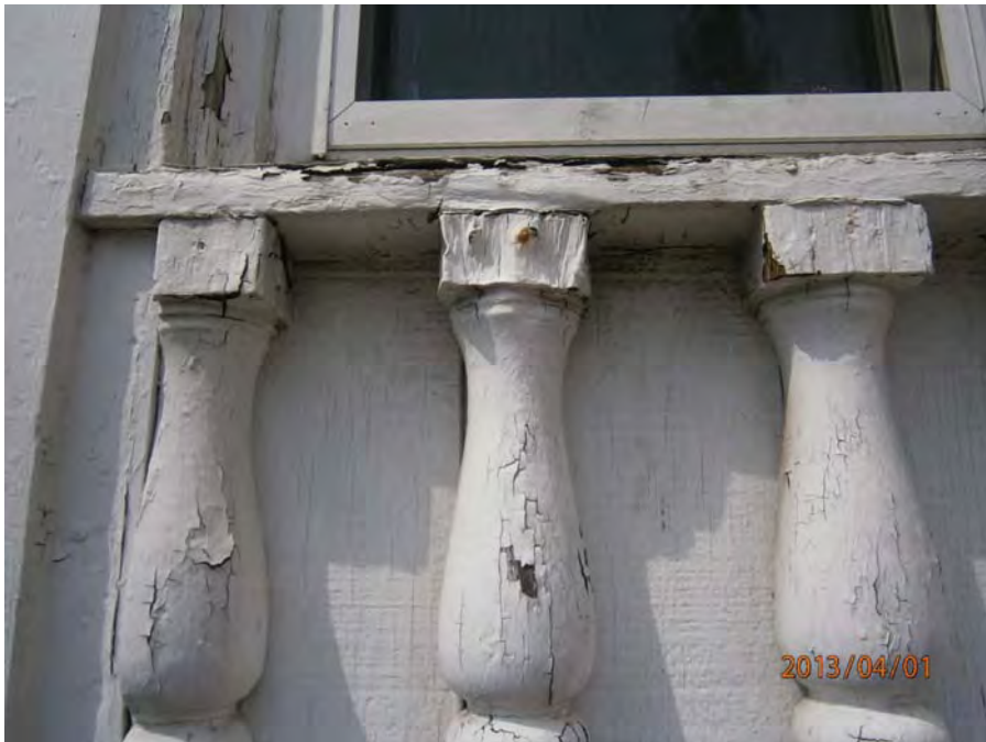
9. Bay window components damaged
