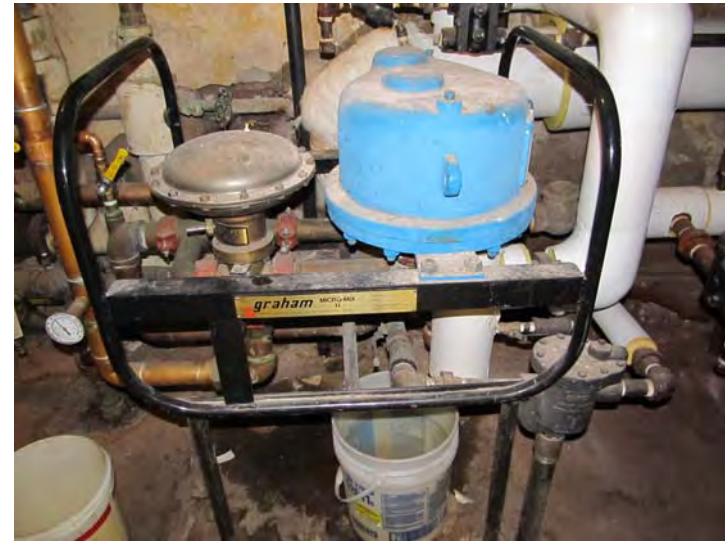
Heat exchanger that utilizes steam from central loop serving hospital campus to produce domestic hot water
