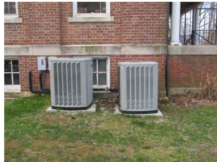
Exterior condenser units work in concert with air handler unit to provide cooling capacity for multi-purpose/dining room
