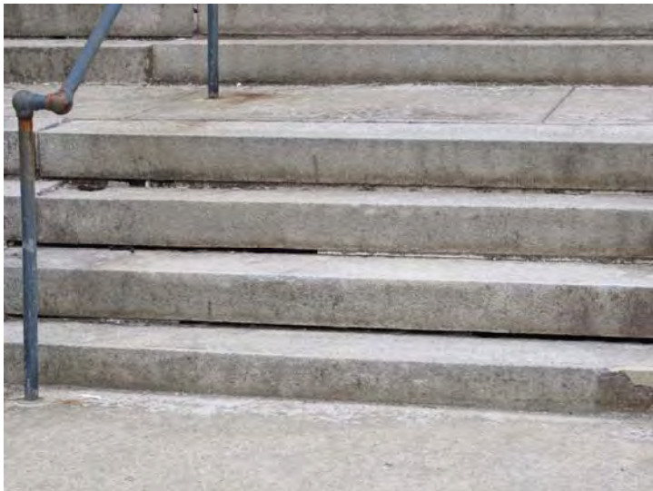
Granite stairs leading to original front entry are in need of re-pointing to prevent water damage
