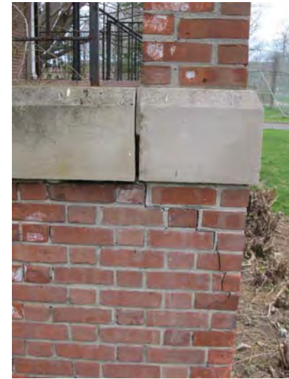
Typical area of mortar loss noted in exterior masonry surface
