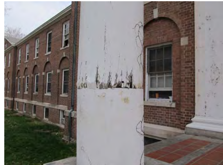
Wood columns at portico of original front entry exhibit rot, deterioration, and past repair efforts
