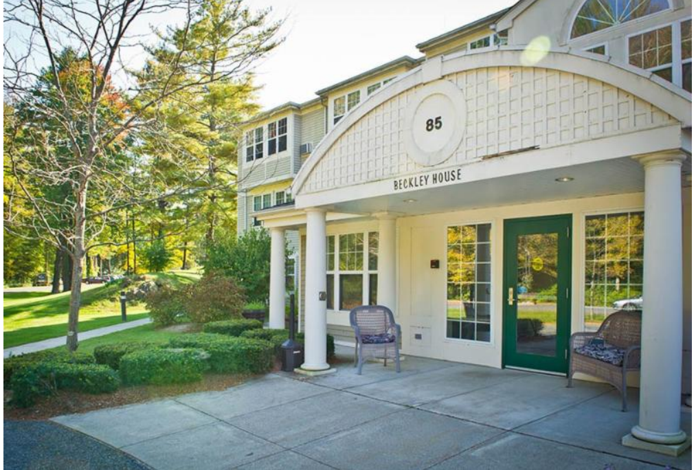
Beckley House in Canaan was funded in part through the Housing Tax Credit Contribution program.
