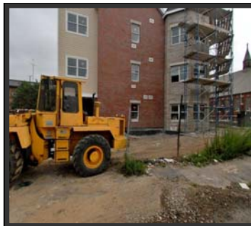
Areyto Apartments Bridgeport 20 units of supportive housing
